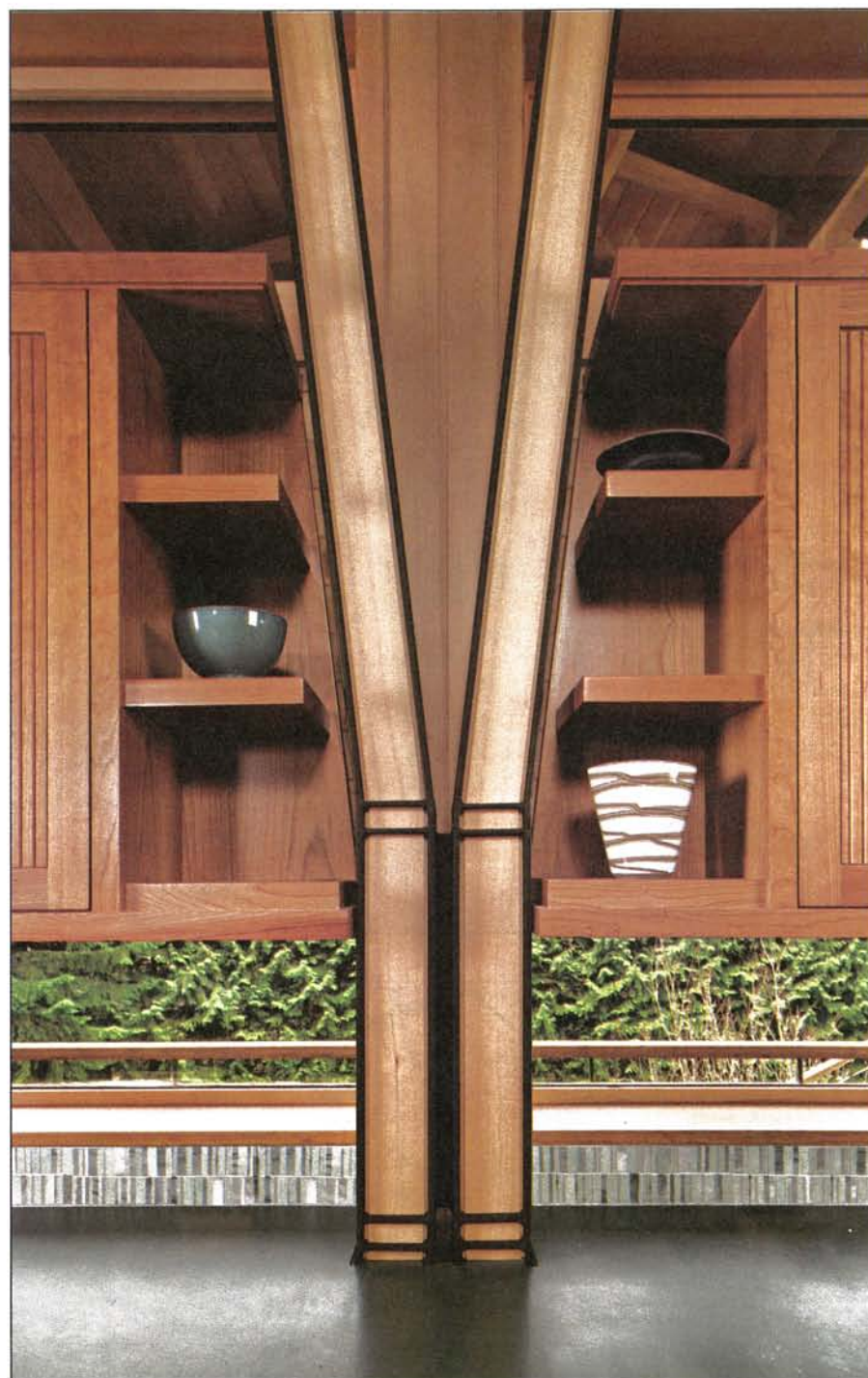
Around the perimeter of the living pavilion, steel posts are formed as two angled columns that meet and then splay apart.
