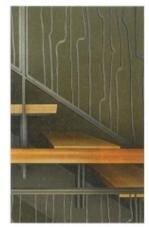
Inside the custom pivot-hinged front door, striking steel and wood stairs have water-jet-cut steel railings with a pattern based on Finne's hand-drawn inkbrush strokes — the same pattern as the front gate, as a matter of fact ... negative on the gate, positive on the stairs.
